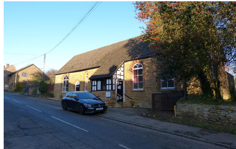
Figure 32 Newnham Village Hall, Church Street.
