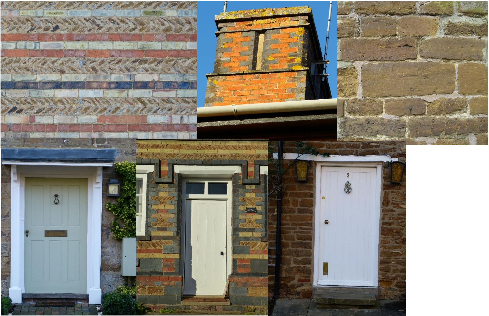
Figure 31 Examples of traditional building materials and finishes, as well as doors within the conservation area.
